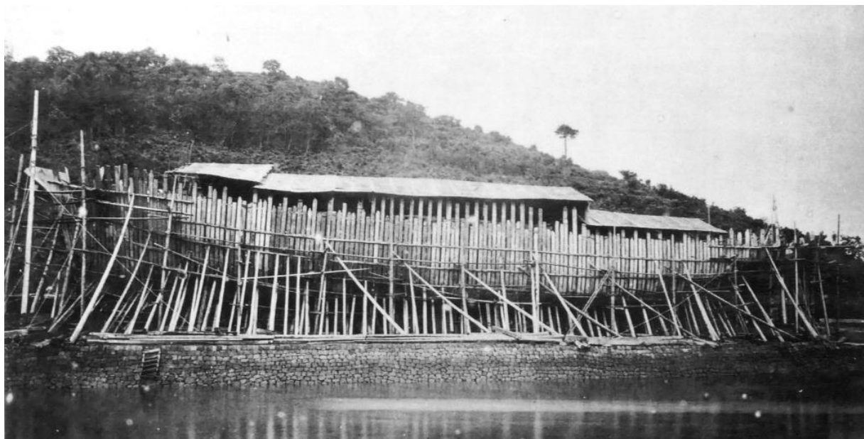
KOSUGE MARU under construction in 1881 (Kosuge Slip Dock).
